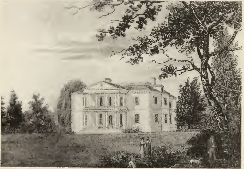
Figure 27. Lansdowne (built 1773, demolished 1854), Governor John Penn's country villa along the Schuylkill River near Philadelphia, Pennsylvania. Engraving from William Birch's Country Seats of...America (Philadelphia, 1808). (Reproduced in Moss, The American Country House , 1990. An original copy of the book is in the possession of The Athenaeum of Philadelphia.)
